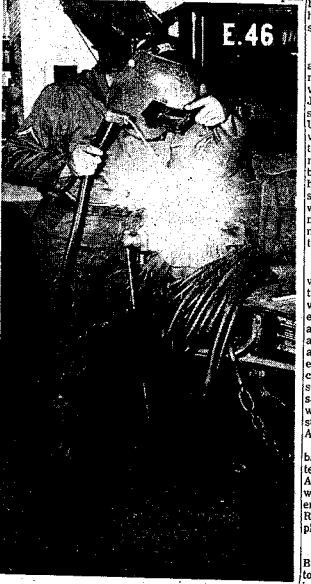
MOBILE WELDER PUT TO USE Used for On-the-Spot Repairs
