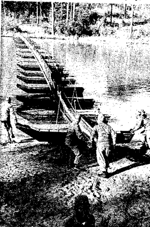
VICTORY POND TRAINING PROJECT Engineers Place Last Section of Foot Bridge
