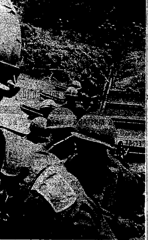
FAST FORD ... A quick construction penton bridge is crossed by members of the 4th Bn., 503rd Abn. Inf. of the 173rd Abn. Bde. The unit was searching for the remains of a Viet Cong battalion which was hit by a B-52 strike earlier. (U.S. Army photo)
